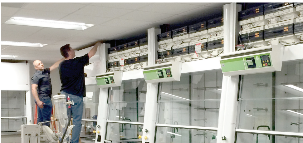
Primary filters being replaced after 5 years of continuous use.
